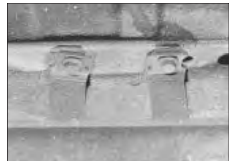
7.9 Fuel tank retaining strap-to-floor bolts
