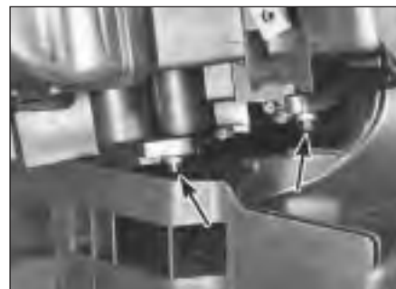
8.6c Control cable connections to flap valves at heater distribution box unit (arrowed)
