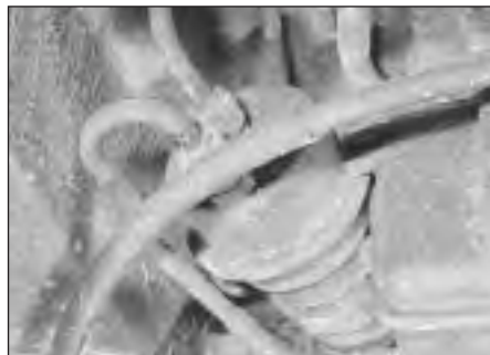
21.1 Fuel accumulator unit location
